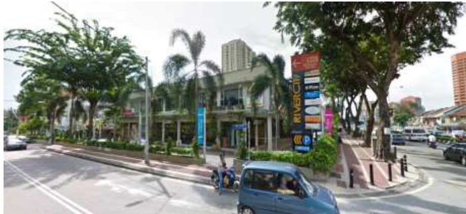
Figure 1: Street view of Riverwalk Village, Jalan Ipoh
